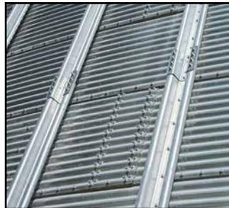
**Sidewall Stiffeners** are among the strongest available to help manage the stress and strain of weather, grain, cables and roof-mounted equipment.
